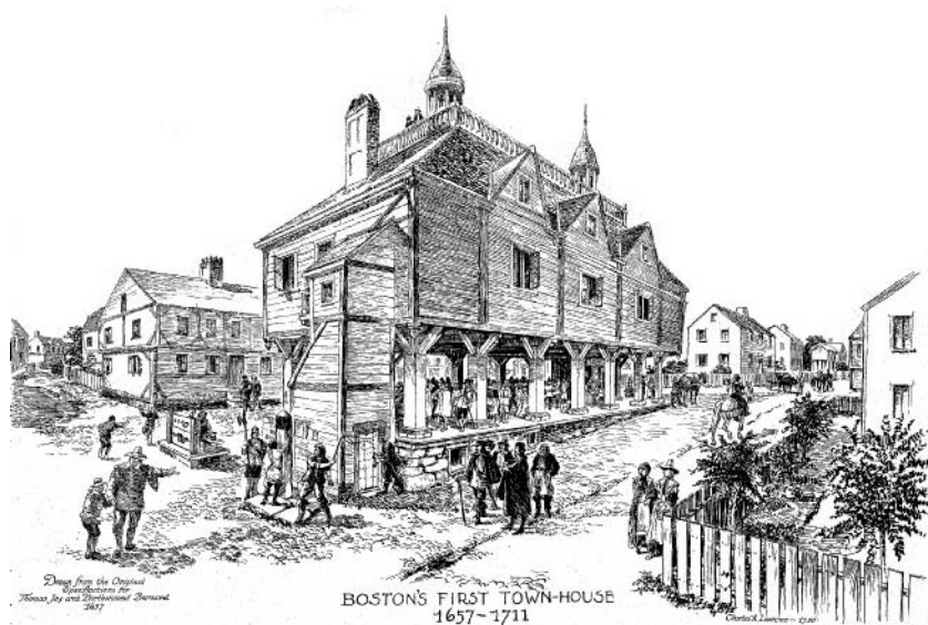
Figure 1.1. Charles Lawrence's 1930 engraving of Boston's Town House, based on architectural drawings, reflects Keayne's plans for the building: a rectangular structure with an open ground floor for merchants to gather, two additional floors for meetings, and a turreted roof. Courtesy of The Bostonian Society/Boston Historical.
